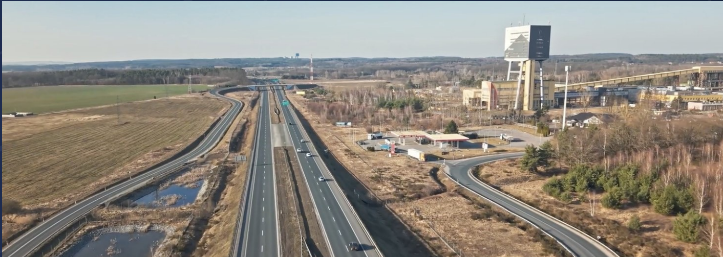
Fully developed road and energy networks in the immediate vicinity of the mine
