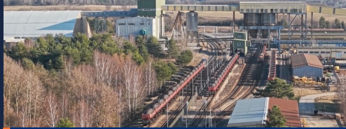
Rail loading yard at the smelter
